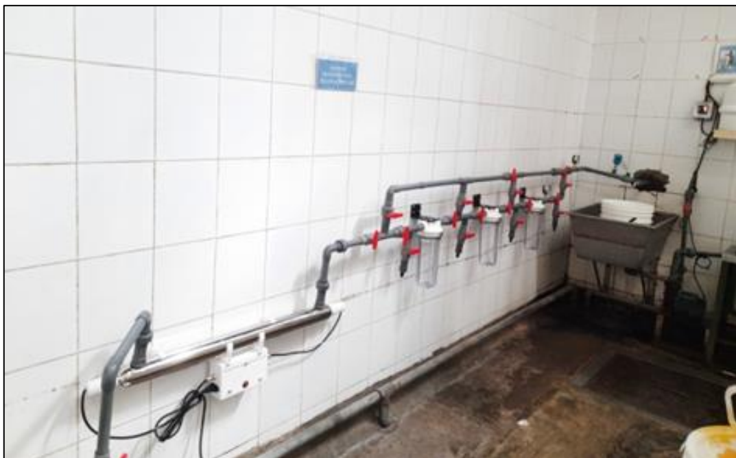
Figure 3. Melt blown filter cartridge and UV-C rays
