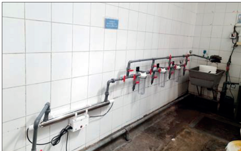
Figure 3. Melt blown filter cartridge and UV-C rays
